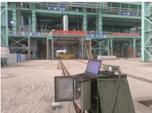
Abb 1: Installation des Dimetix Sensors
