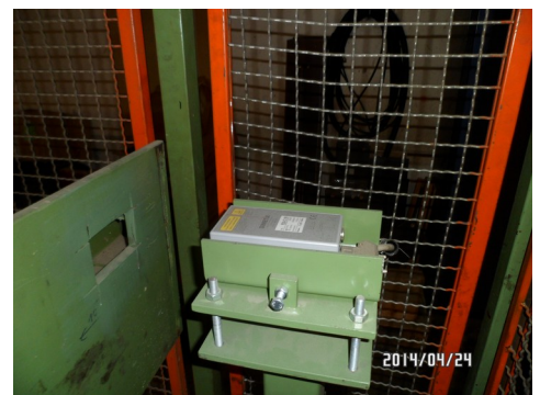
Fig 2: Installation of Sensor
